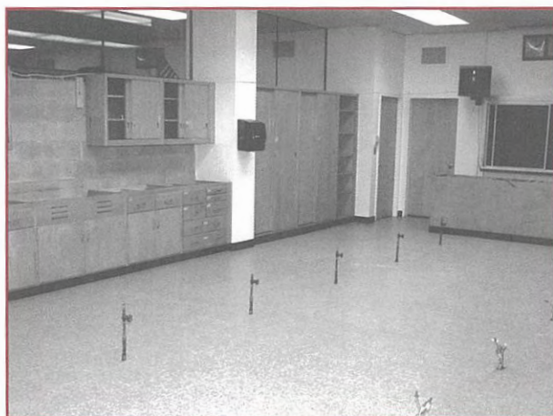
The physics laboratory shown above, as well as the biology and chemistry labs, are being completely renovated this summer as part of a grant from Empire State Development Co. Photo by Alex Malecki
